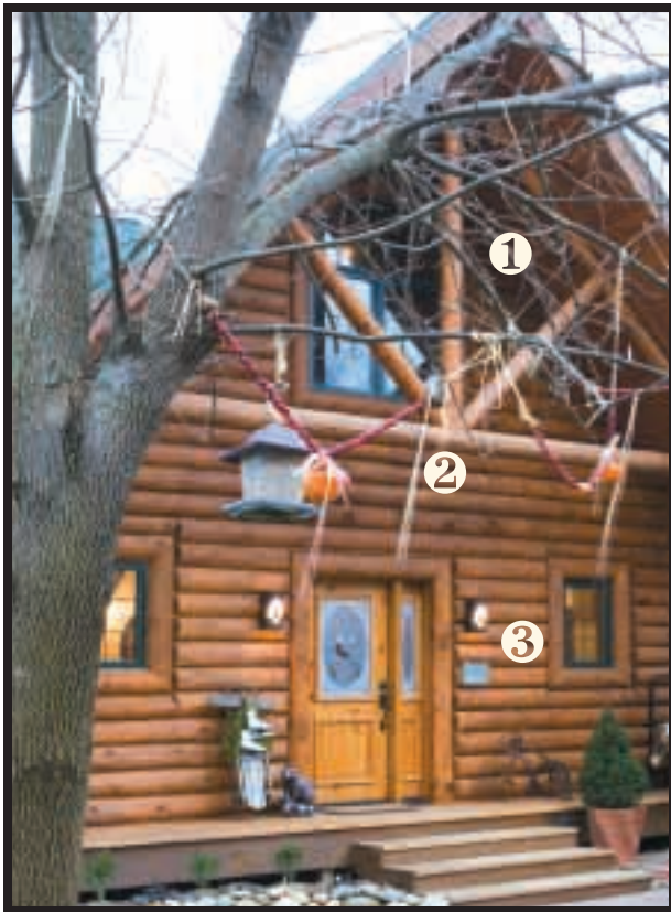
① Open gable porch ② Log tie beam with king post & diagonals ③ Round log four-sided window trim
