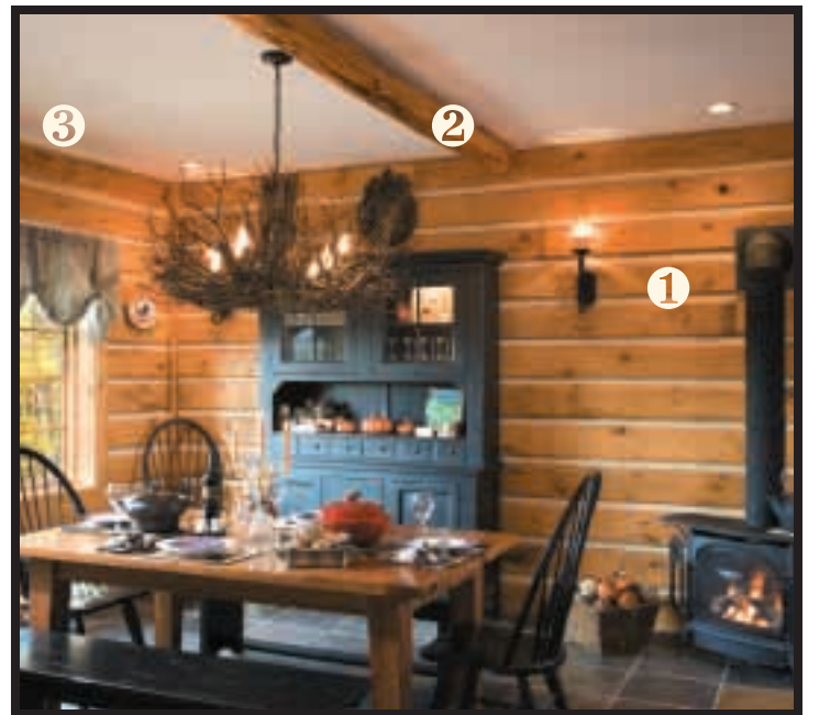
Right 1 Interior timber log with chinking 2 Log rafter on flat ceiling 3 Drywall ceiling
