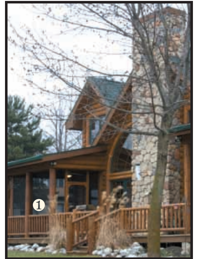
① Shed screen porch
