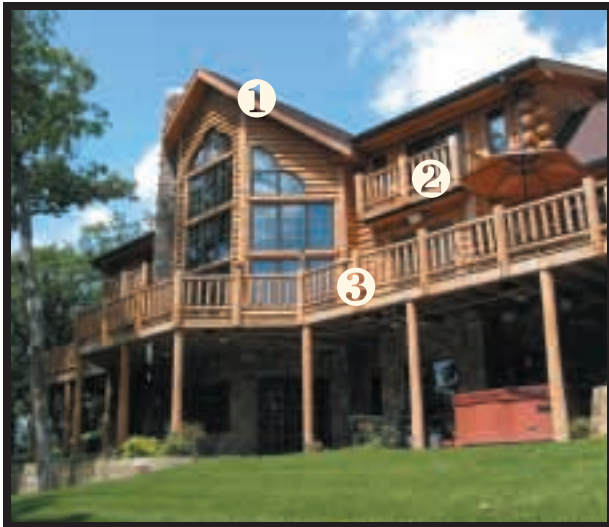
1 Clipped center gable 2 Log balcony 3 Elevated deck
