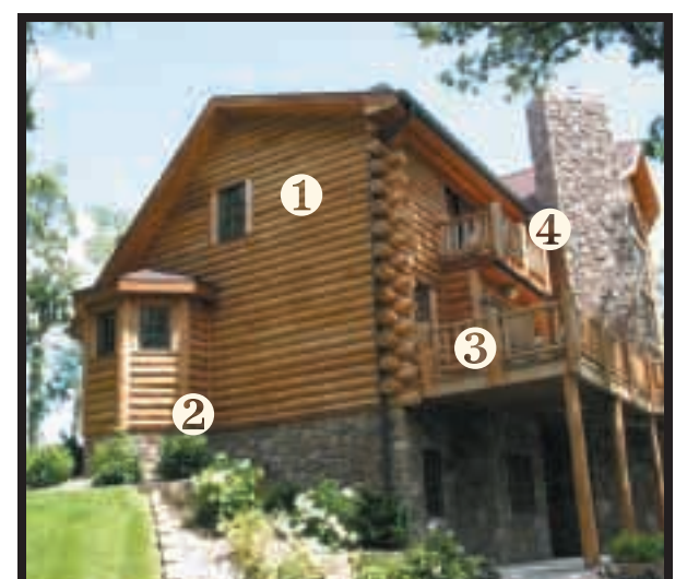
① Shed dormer to end of house ② Bumpout ③ Elevated deck ④ Balcony
