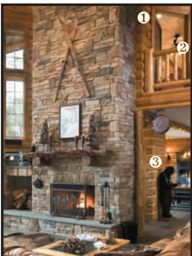
1 Interior round half log 2 Standard cedar safety rail 3 Interior timber log with chinking
