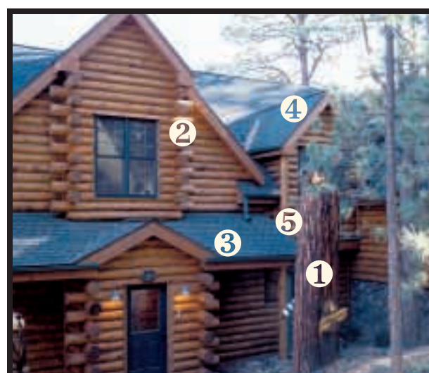
① Bear carved in tree ② Bumpout ③ Roof "eye-brow" ④ Gable dormer ⑤ Vertical post corner
