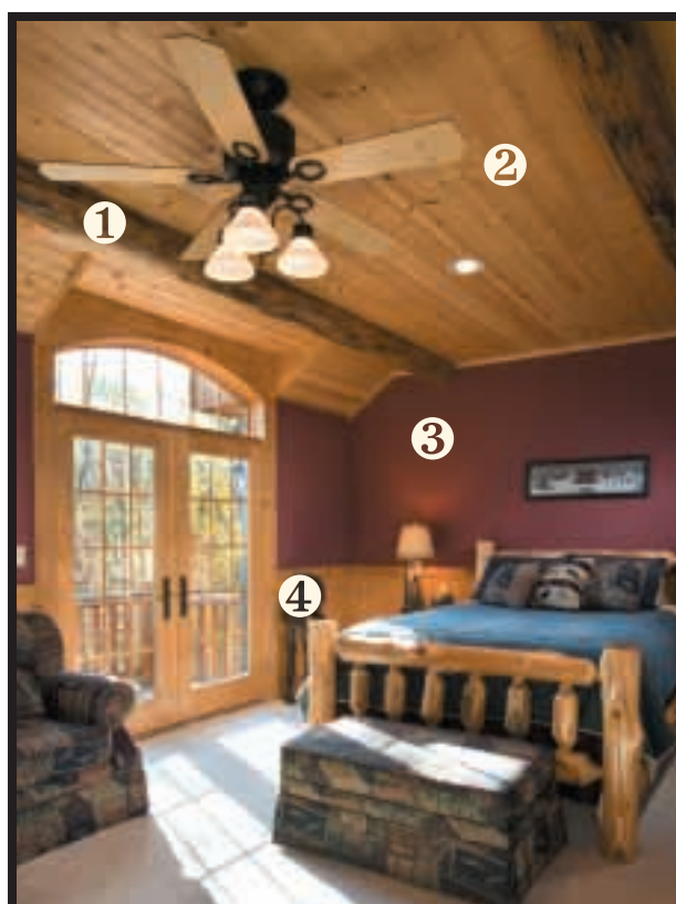
1 Log rafter on flat ceiling 2 Knotty pine on flat ceiling 3 Painted wall 4 Knotty pine wainscoting
