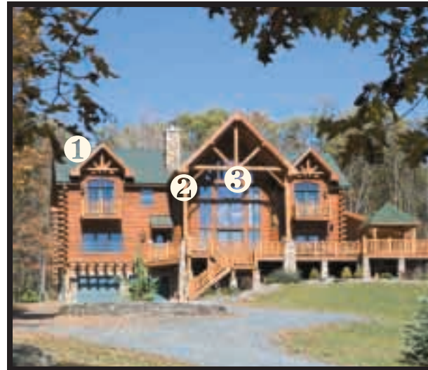
1 Gable bumpup 2 Open gable porch 3 Log tie beam with king post & diagonals
