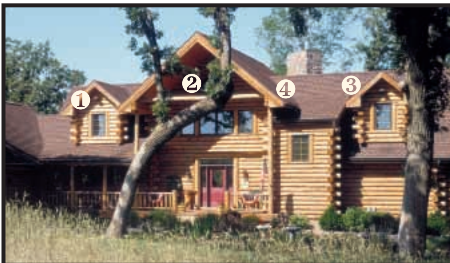
1 Gable dormer 2 Open gable porch 3 Boxed eaves 4 Center section higher than wing roof line
