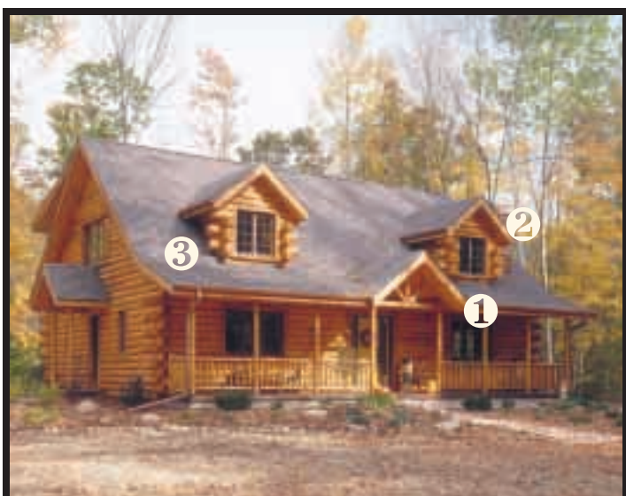
1 Shed porch with flat ceiling 2 Gable dormer combined with open gable porch 3 Raked eaves
