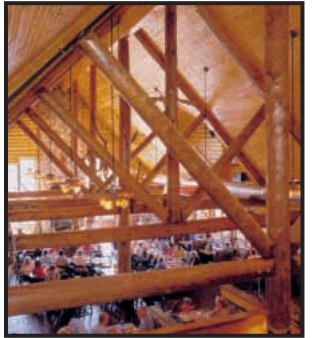
Log trusses framing the diners below
