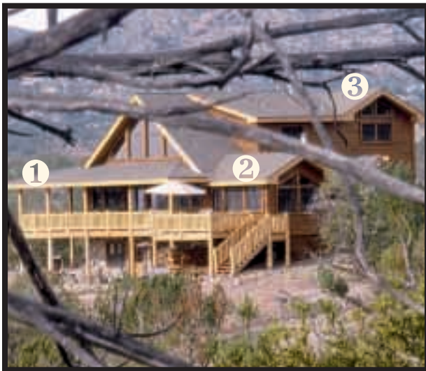
① Shed porch ② Sunroom ③ Blended shed dormer into gable section
