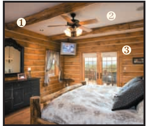
1 Log rafter on flat ceiling 2 Drywall ceiling 3 Interior timber log with chinking
